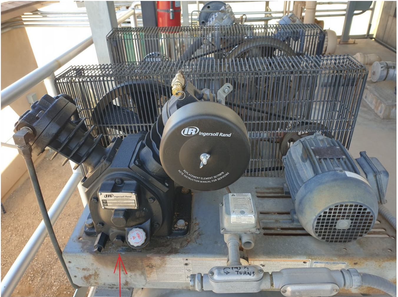
New Ingersoll Rand Duplex air compressor head assembly for water plant filtration system.
