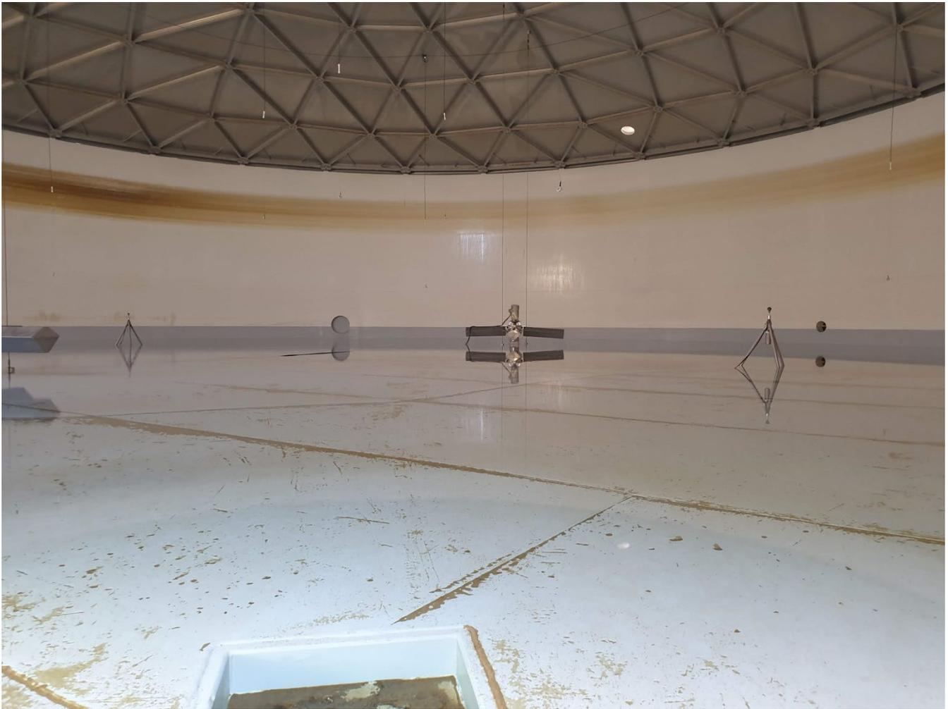
**Interior photo of 2.4 MG Tank. Minor blistering of epoxy coating was noted on the floor of the tank. Arrangements will be made to repair/replace coating on noted areas later this year (Fall 2023) after the peak summer demand.**
