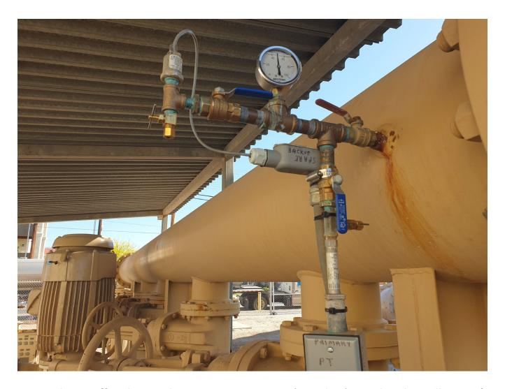
Water Plant staff and Controls Systems Engineering (*Eric Blom*) completed installation of new <u>dual pressure transducer manifold</u> with secondary backup transducer at distribution pump station.
