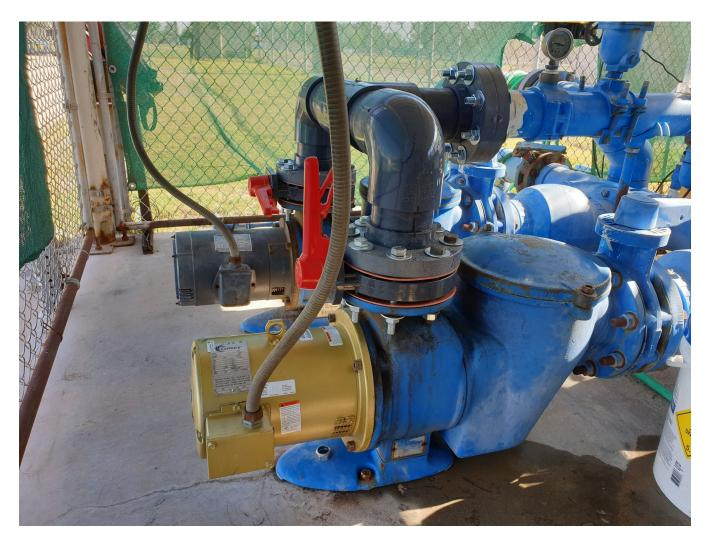
Staff completed discharge valves and piping replacement, as well as installation of newly reconditioned South Recirculation Pump (shown above in gold color) at Gene Layton Memorial Pool in preparation for annual Public Health Inspection.
