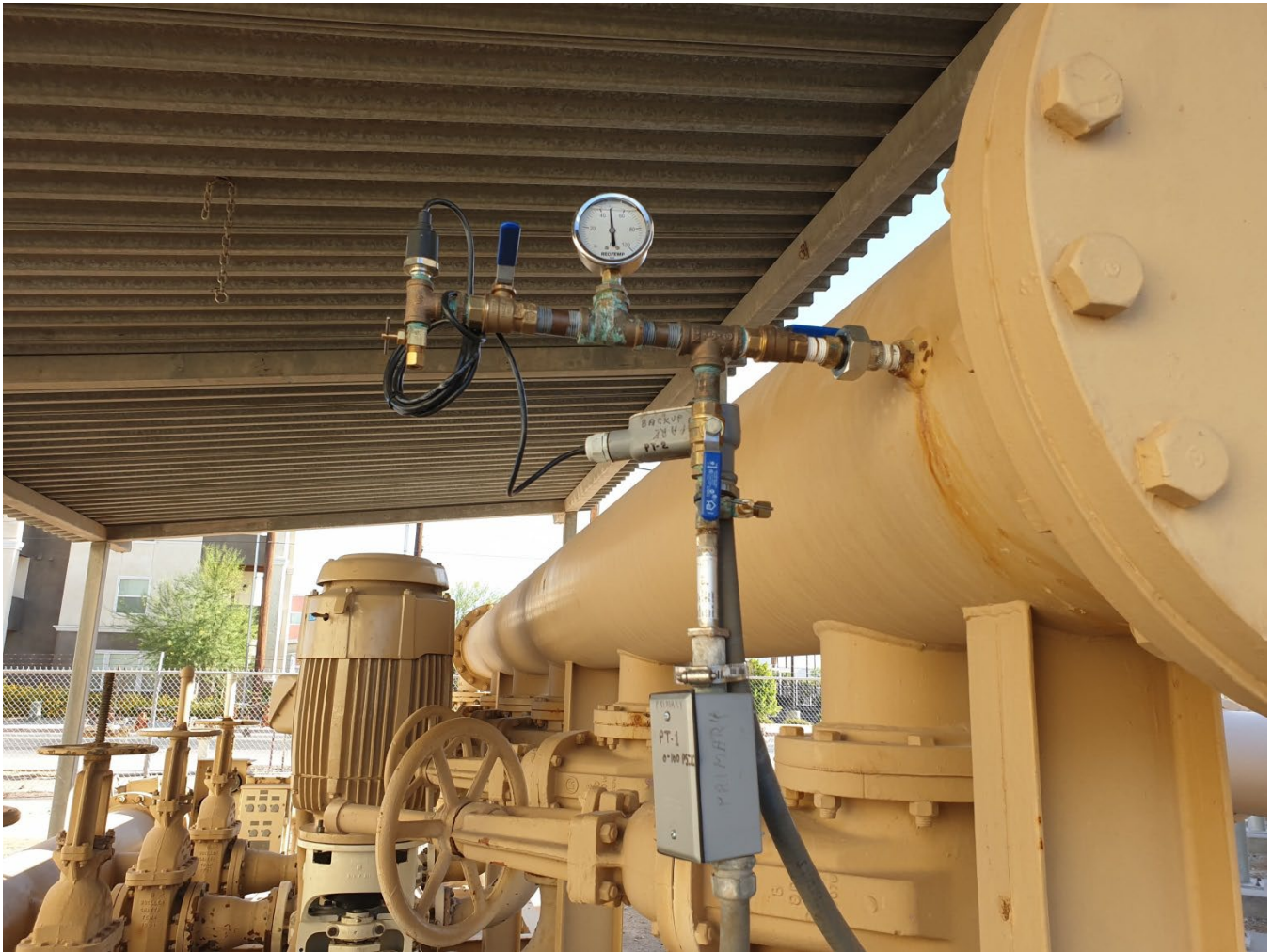
New dual distribution pressure transducer manifold installed at booster pump station.
