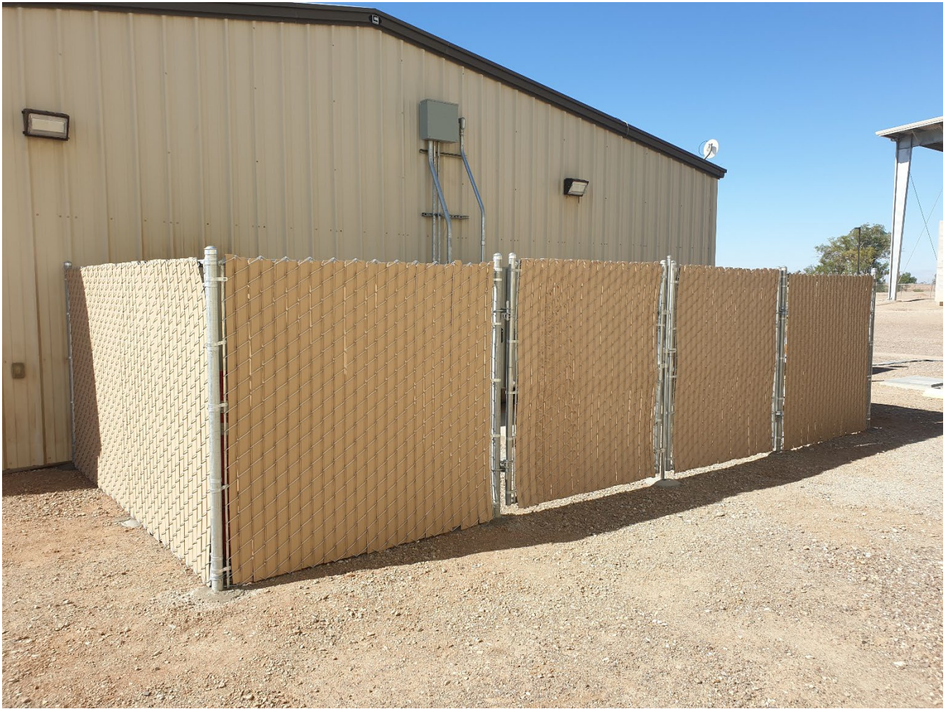
New privacy security fencing along north side of water plant.
