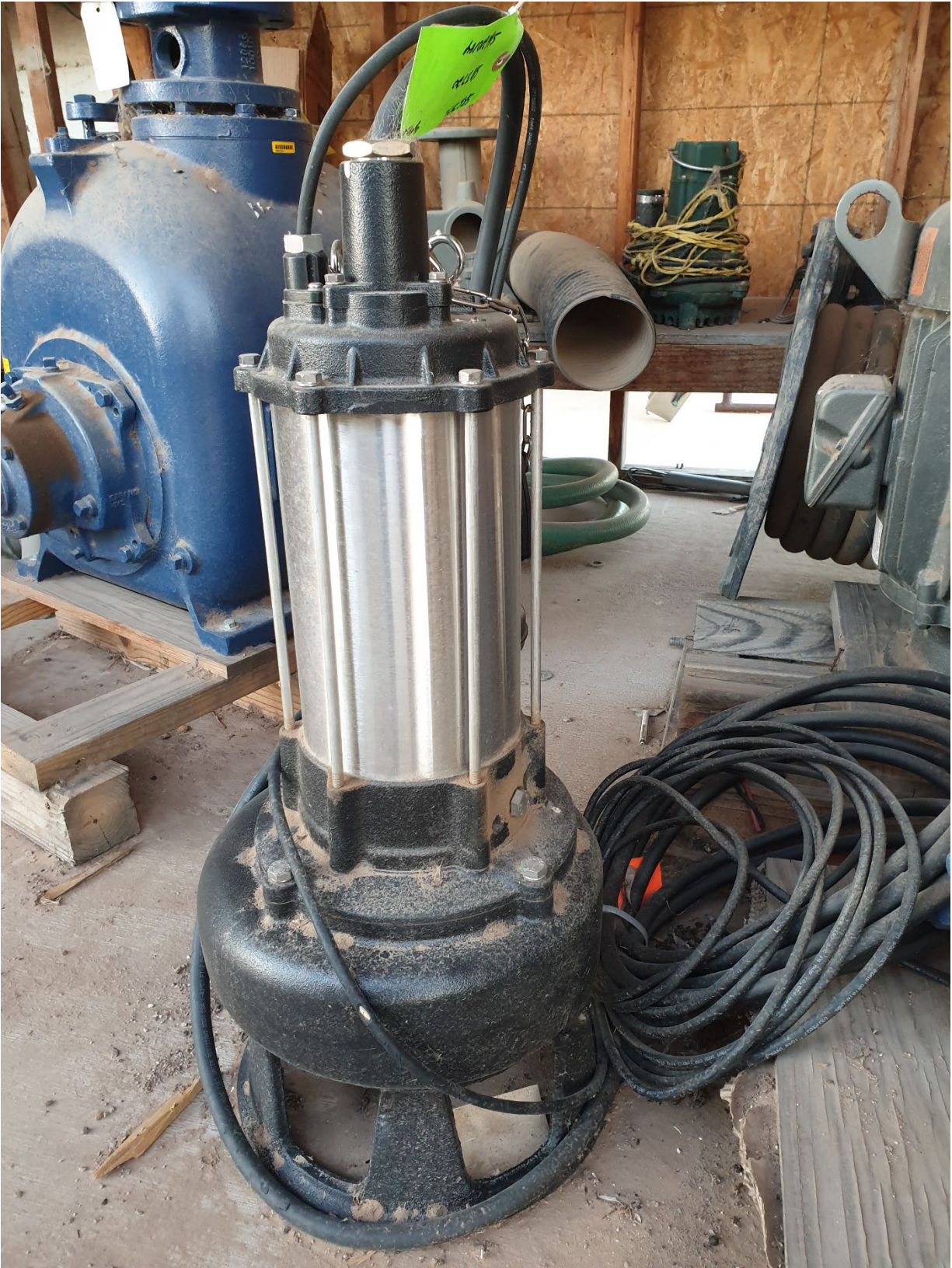
New Landia chopper pump unit installed at SE clarifier basin.
