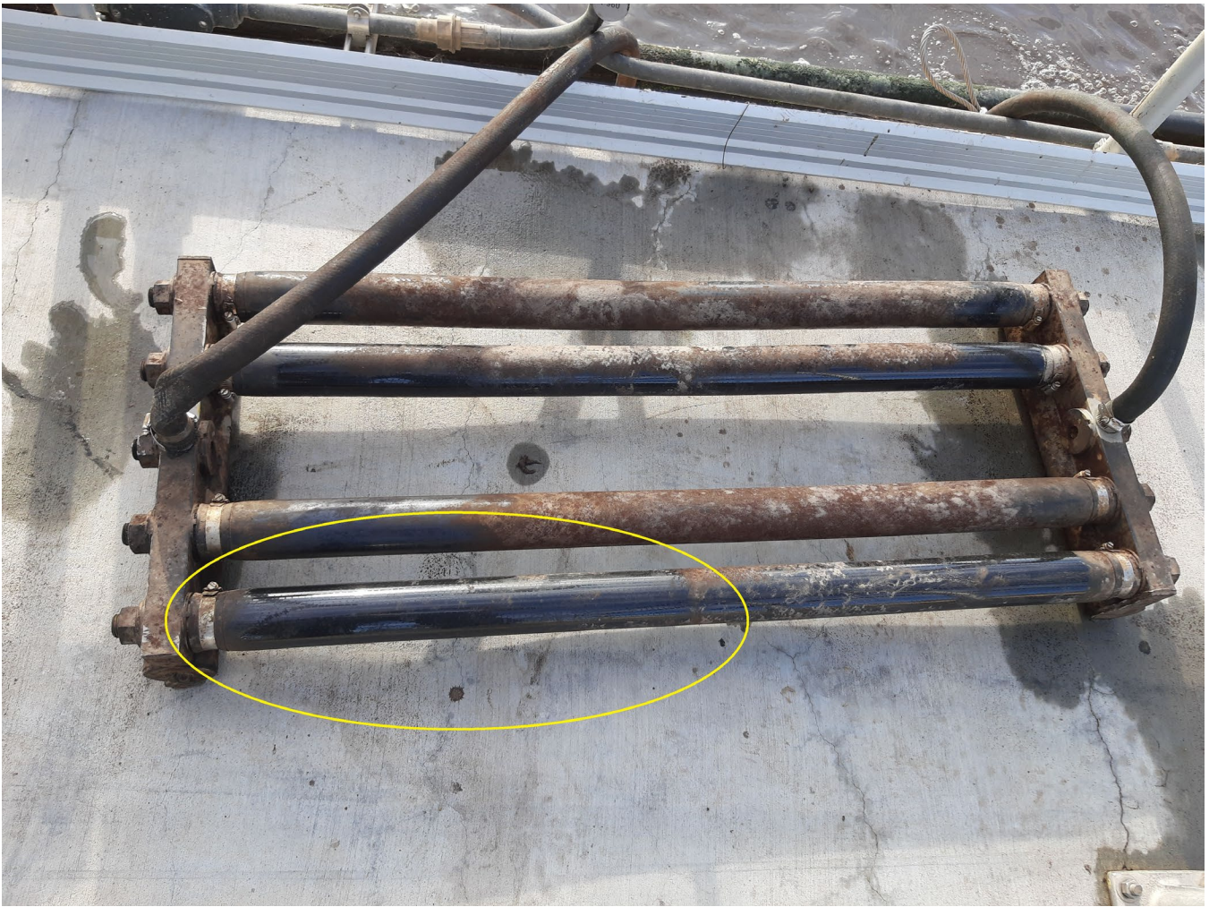
Membrane replacement work on Biolac aeration diffuser rack assembly.
