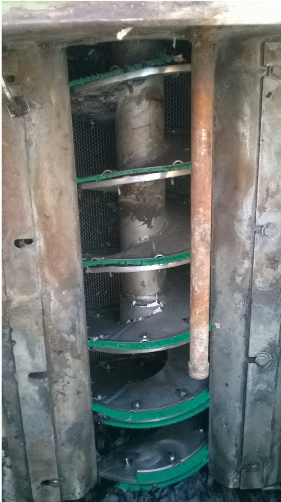
Close-up view of new headworks auger screen brush assembly
