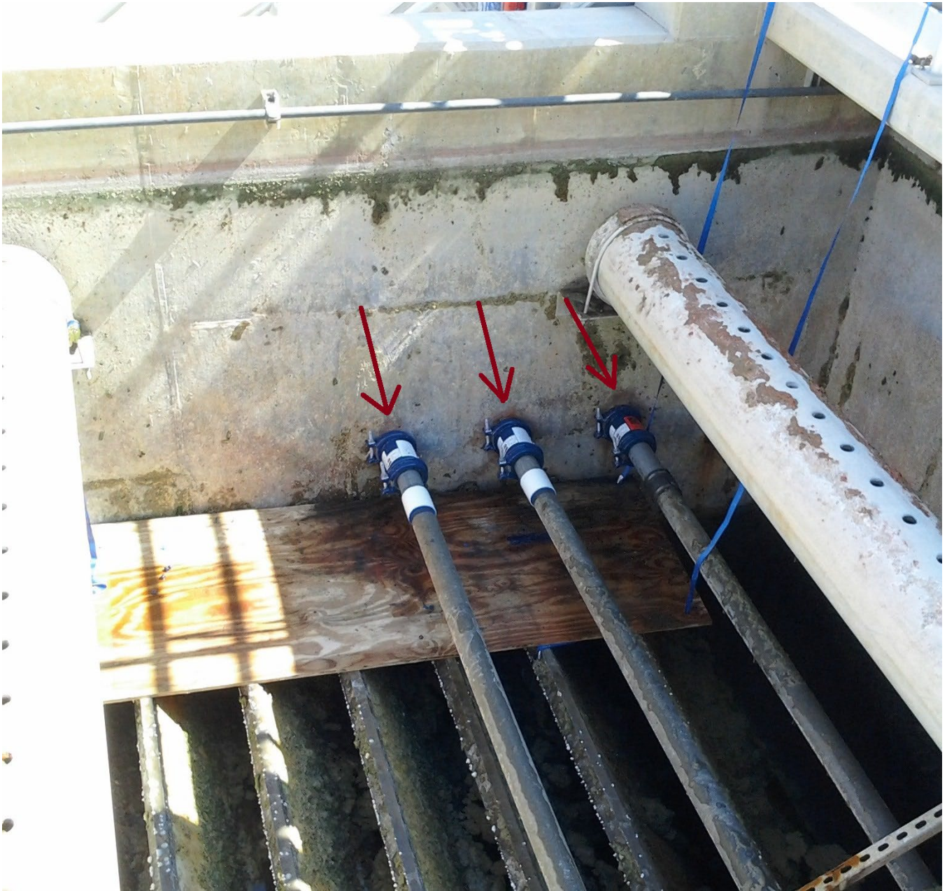
North upflow clarifier basin compression couplings replaced.
