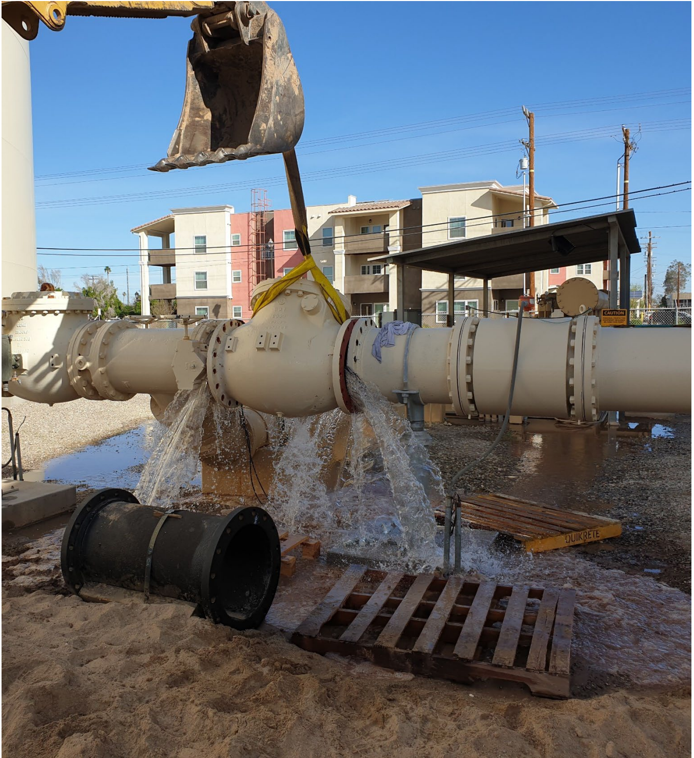
Removal of discharge check valve from 2.4 MG Storage Tank
