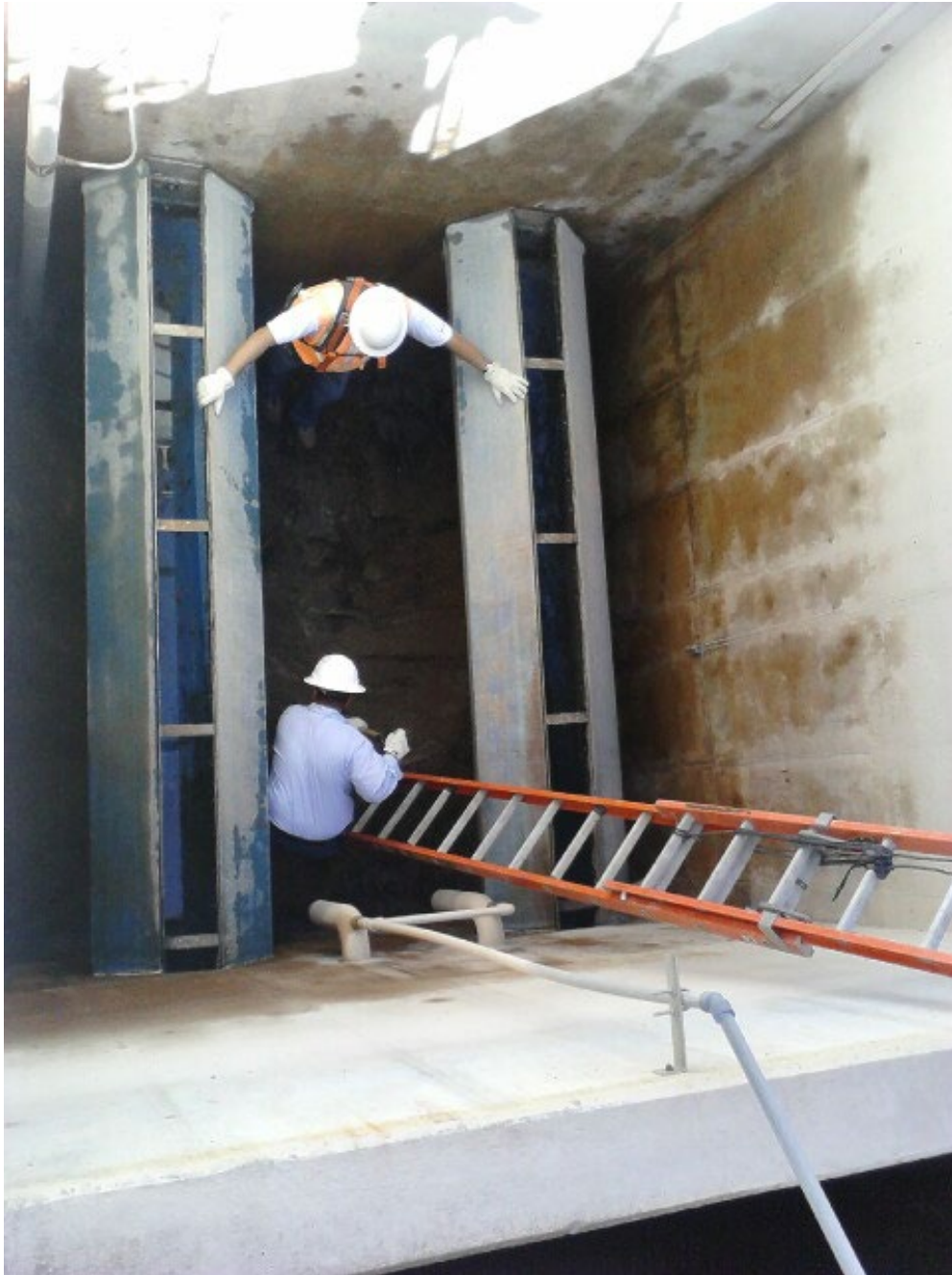
Water plant staff inspecting filter media bed in Filter Cell #1
