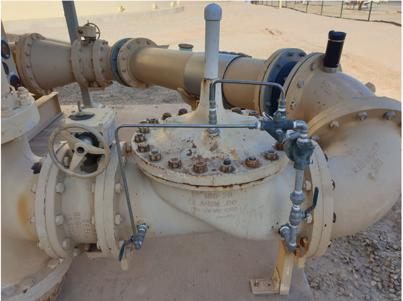
Cla-Val technicians rebuilt and tested the 12" pressure relief valve on the discharge side of the distribution pump station.
