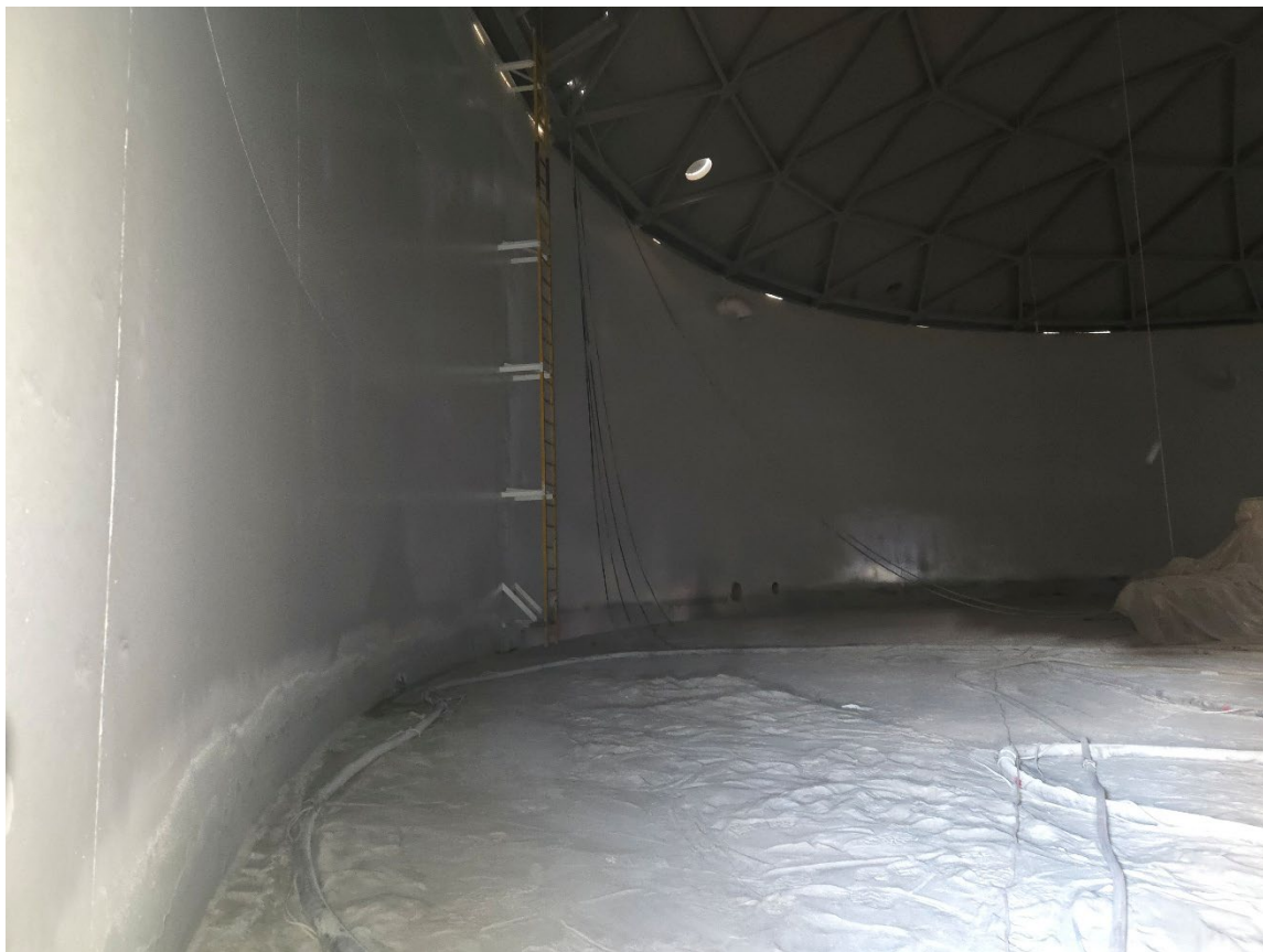
Interior view of South Side Wall after sandblasting
