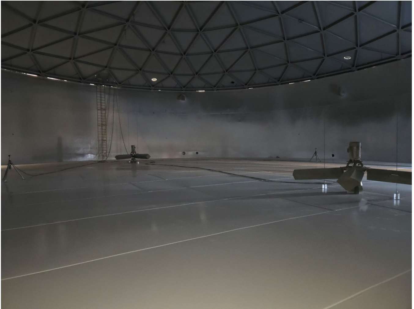
Interior view of complete recoating work inside 2.4 MG storage tank
