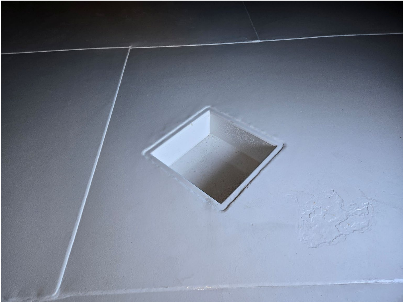
Close-up view of coating work on drain sump inside 2.4 MG storage tank
