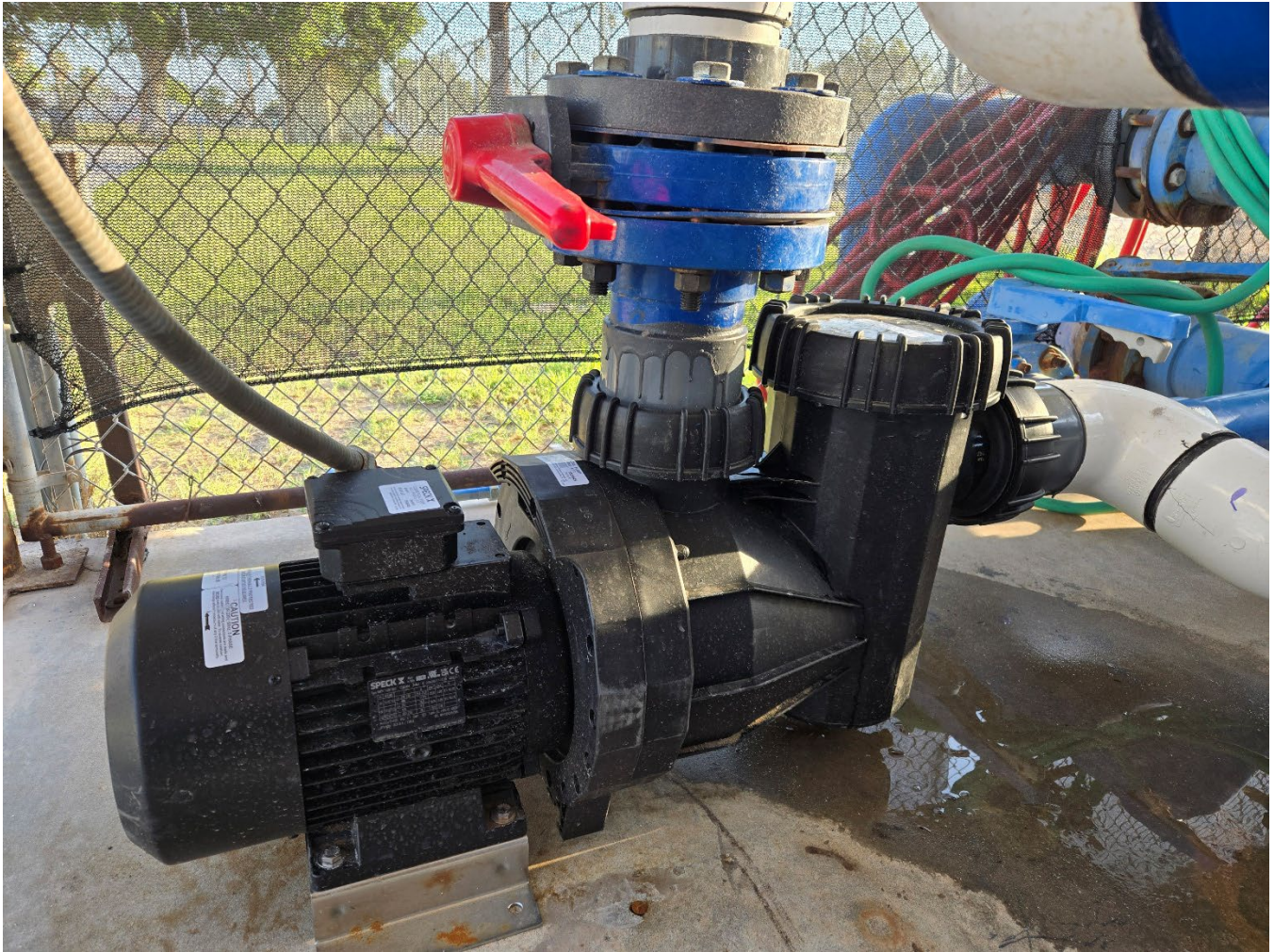
New Pentair VFD Pool Recirculation Pump #1
