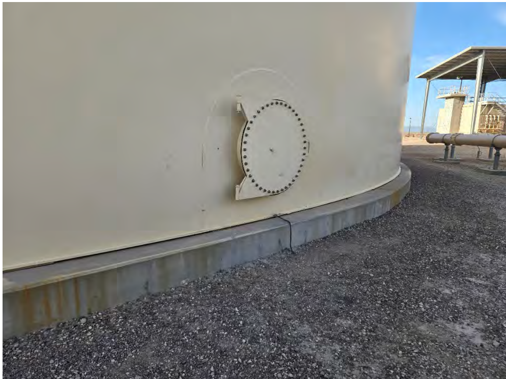
No signs of leakage at northern base of 2.4 MG Tank
