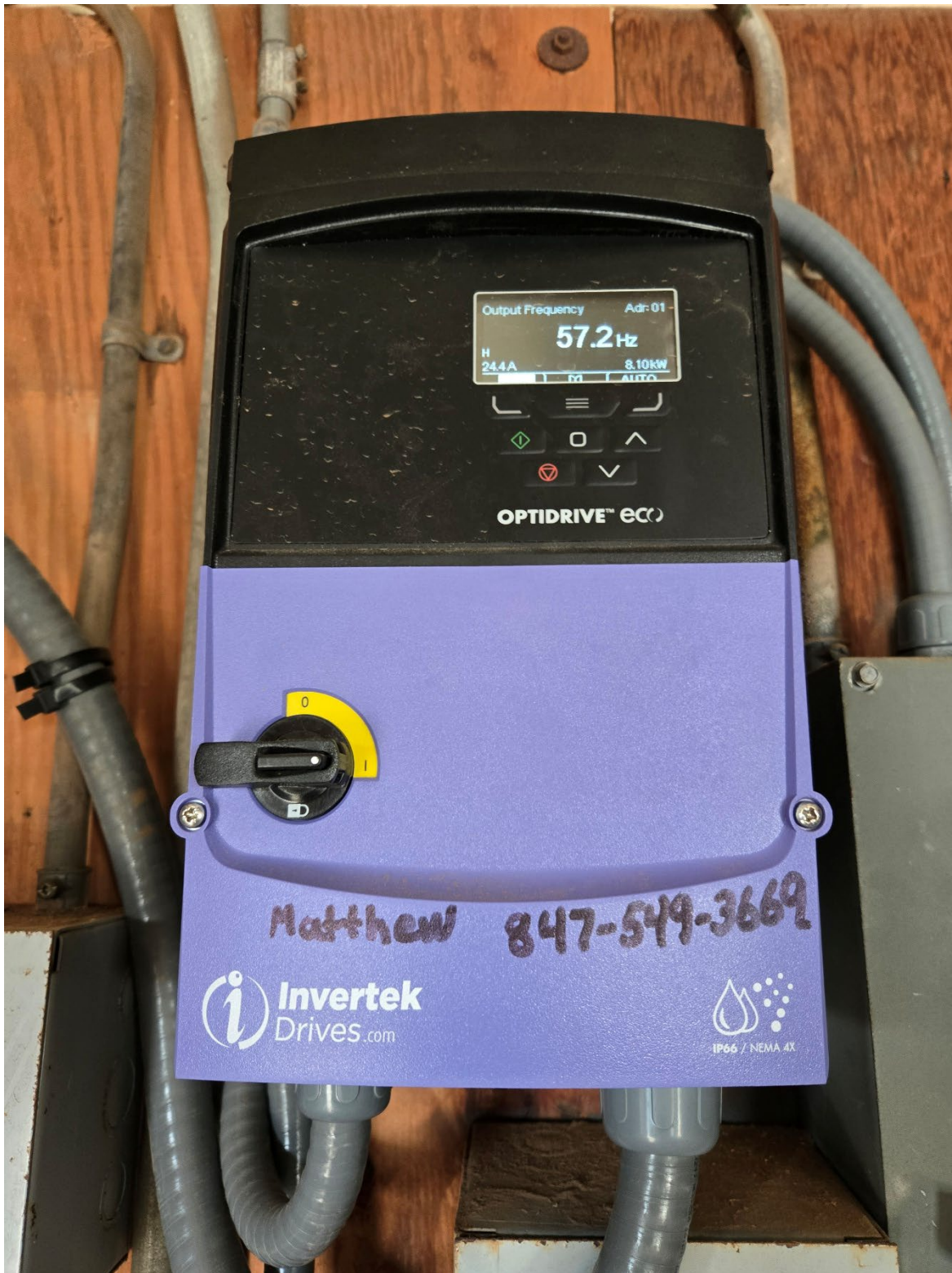
New Variable Frequency Drive pump speed controller for Pentair Pumps
