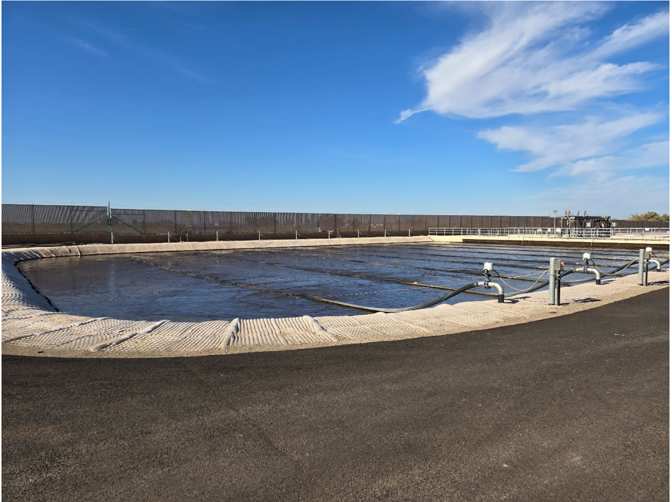
View looking south across Biolac aeration basin shows aeration diffuser chains scheduled to be replaced by EDI Inc.
