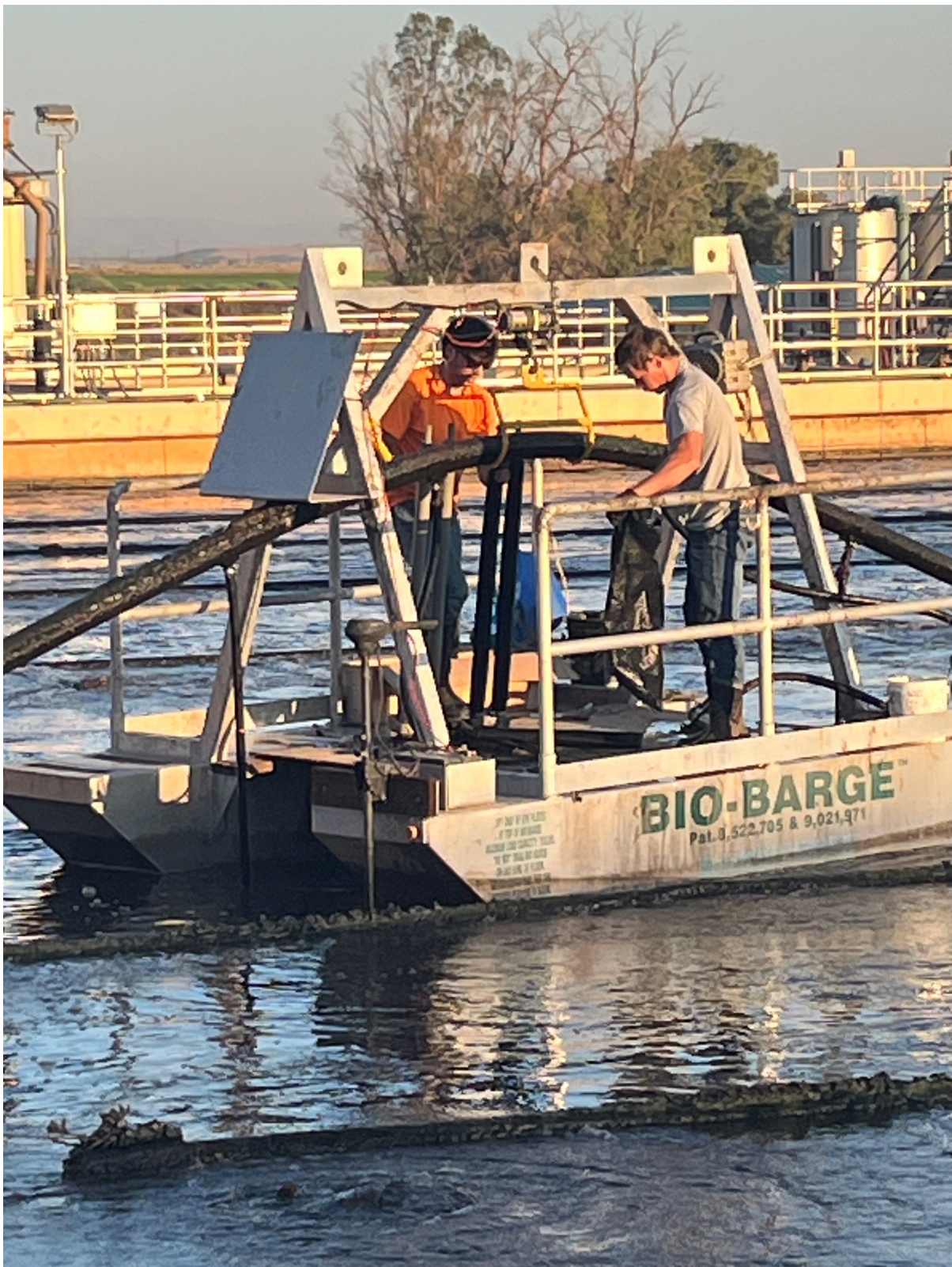
EDI work crew pulling up an aeration diffuser rake assembly
