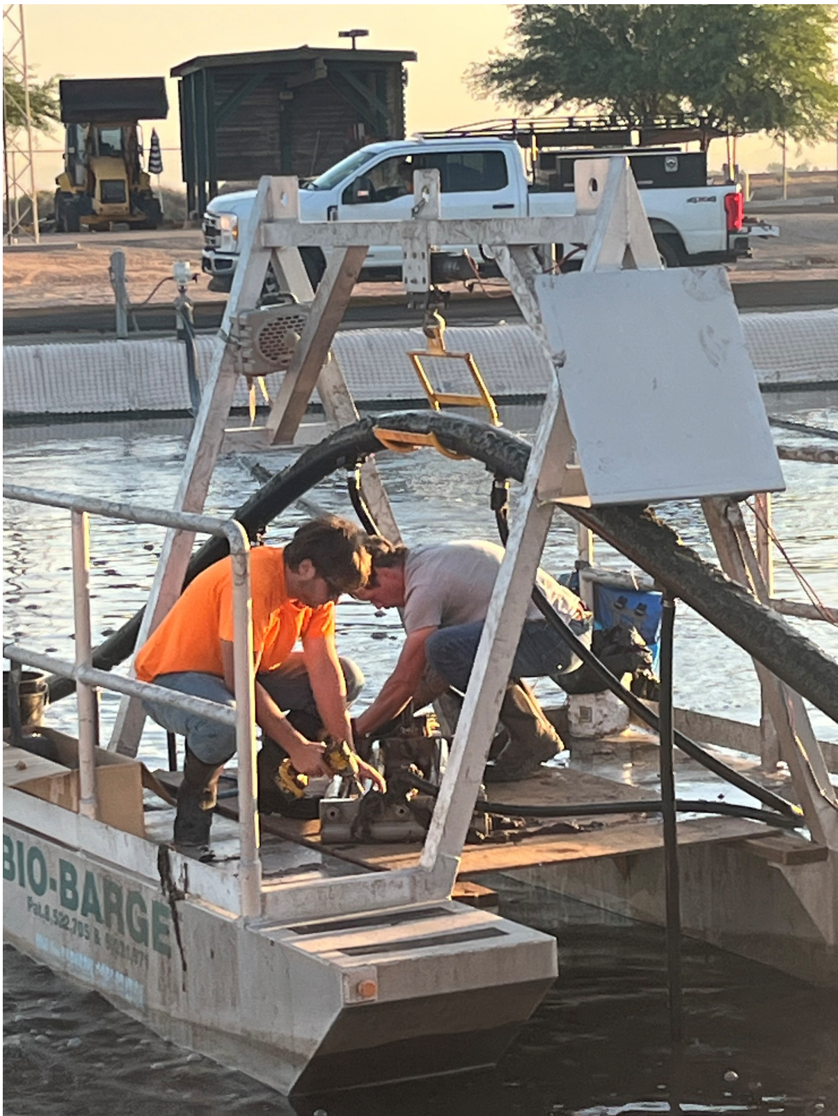
EDI work crew replacing membrane on aeration diffuser rake assembly
