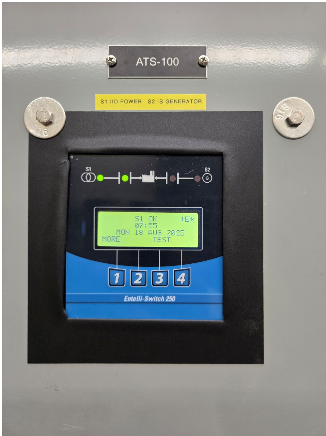
Water plant emergency standby generator automatic transfer switch
