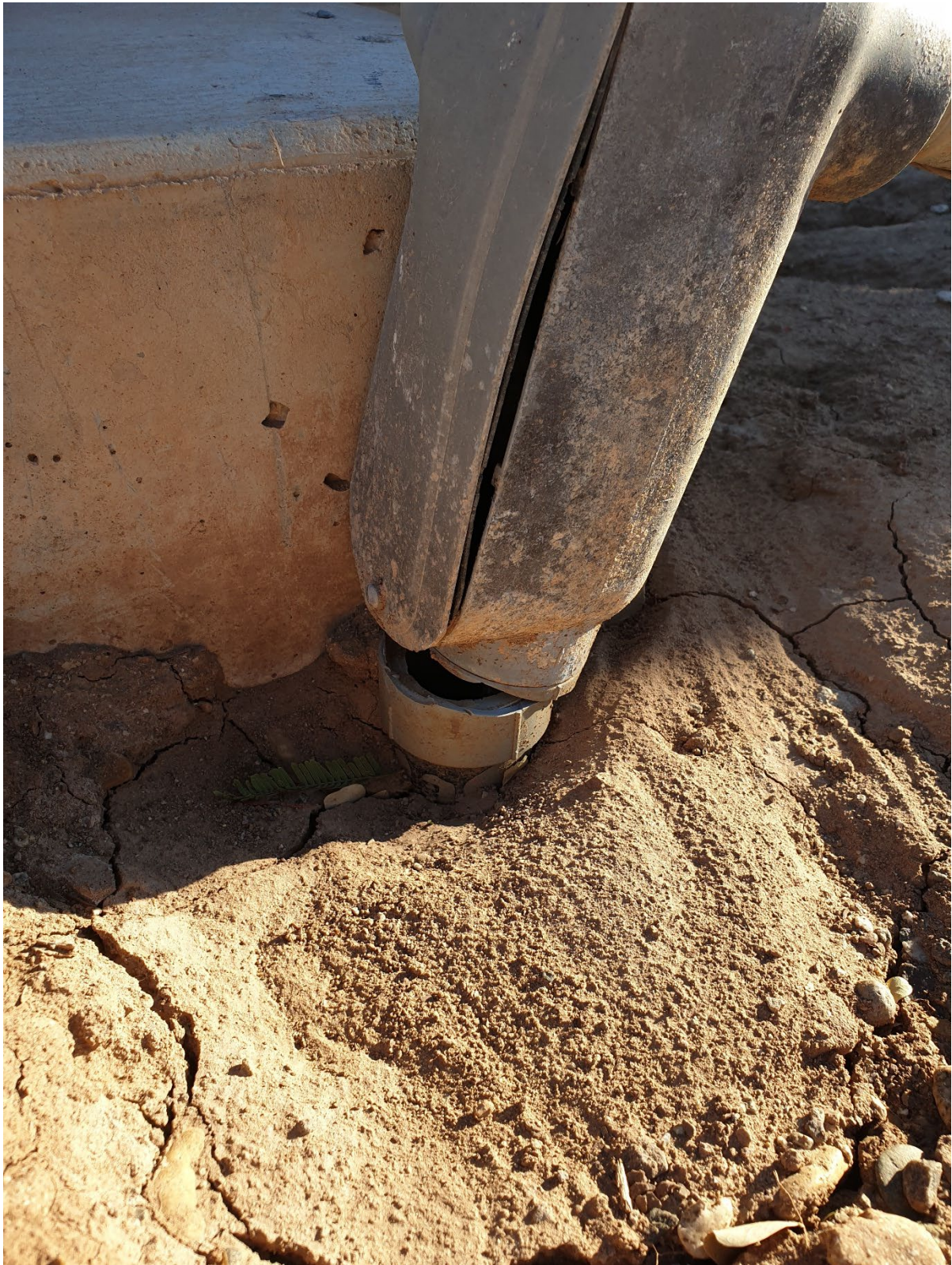
Damaged cable junction box at raw water pump station
