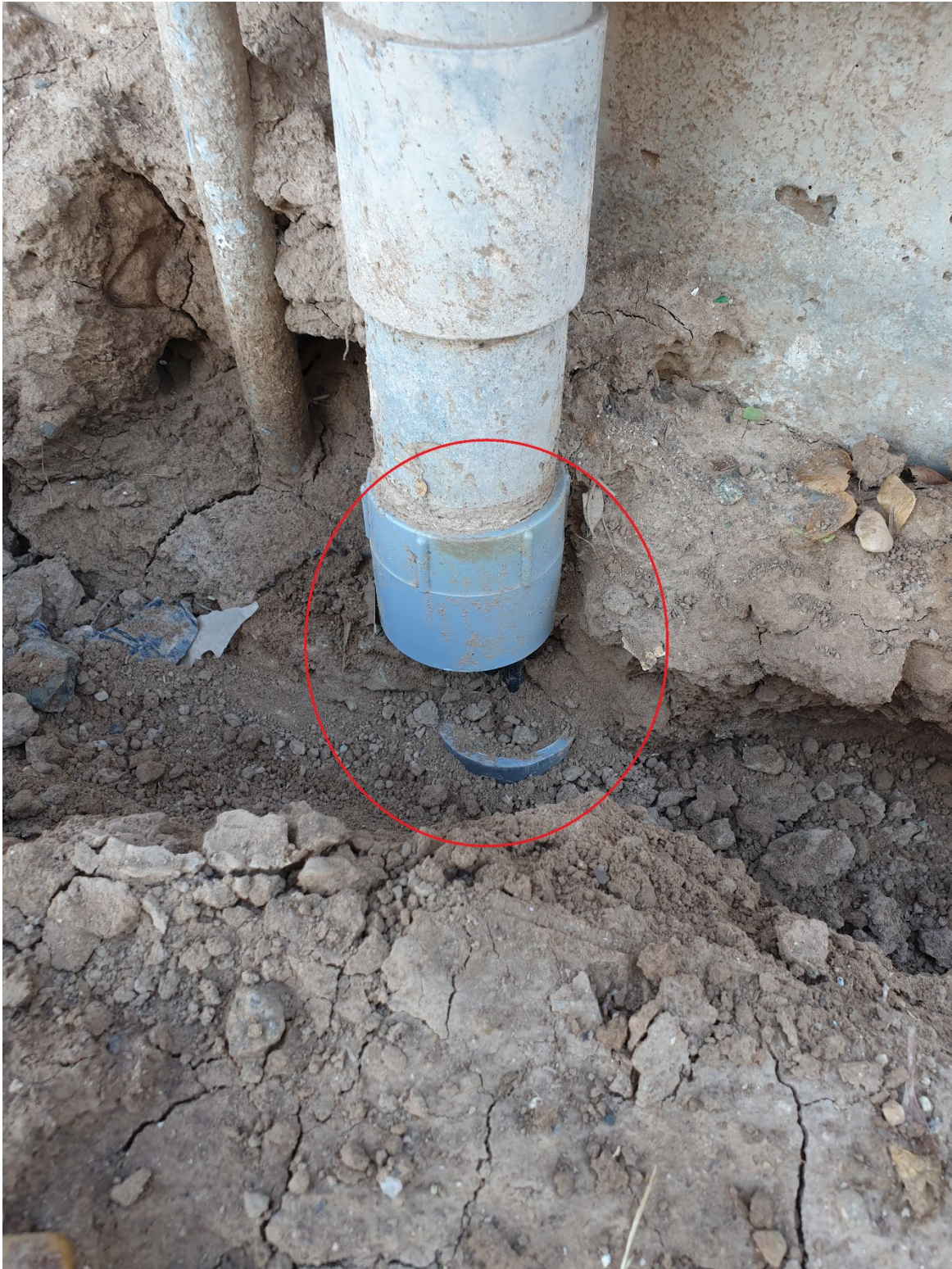
Electrical conduit break with exposed wiring
