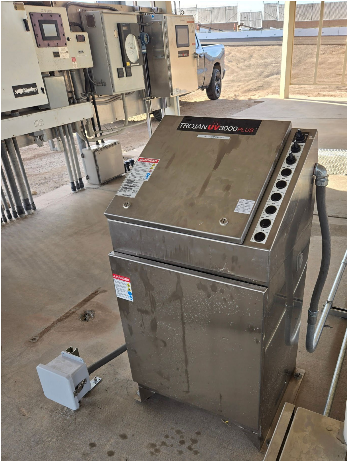
New hydraulic wiper control cabinet for banks 1 & 2
