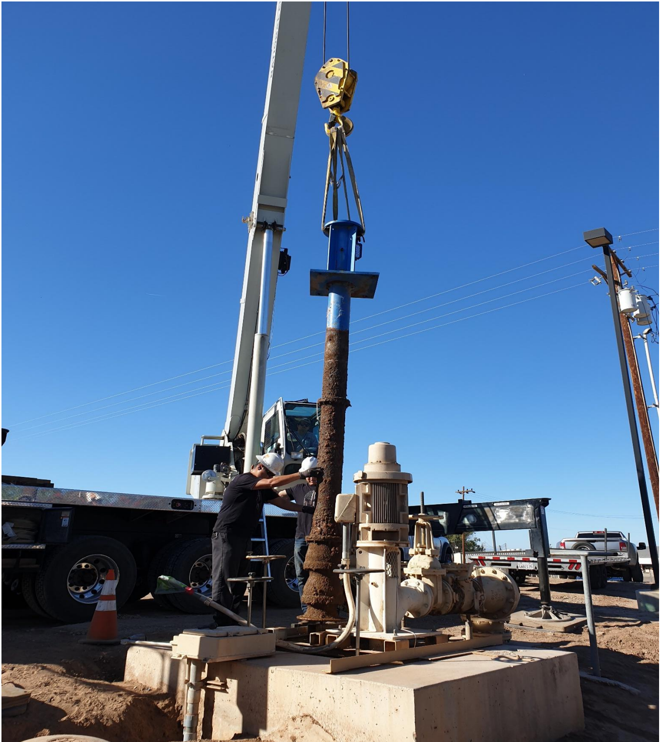
(DXP & Craig's Crane removing the 7-year-old pump & motor)
