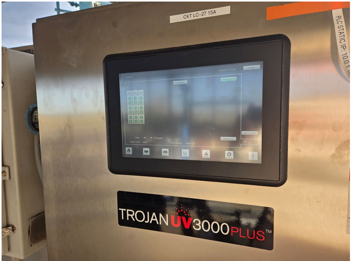
New Trojan UV 3000 Human Machine Interface (HMI) and control center
