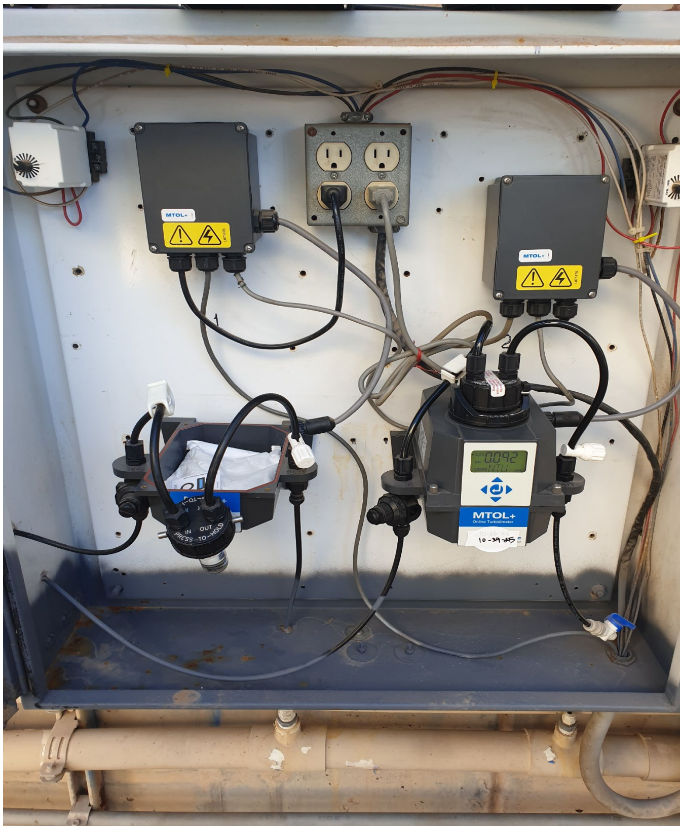
(Turbidity meters 1 & 2) (#1 was replaced with our backup after a bulb failure)
