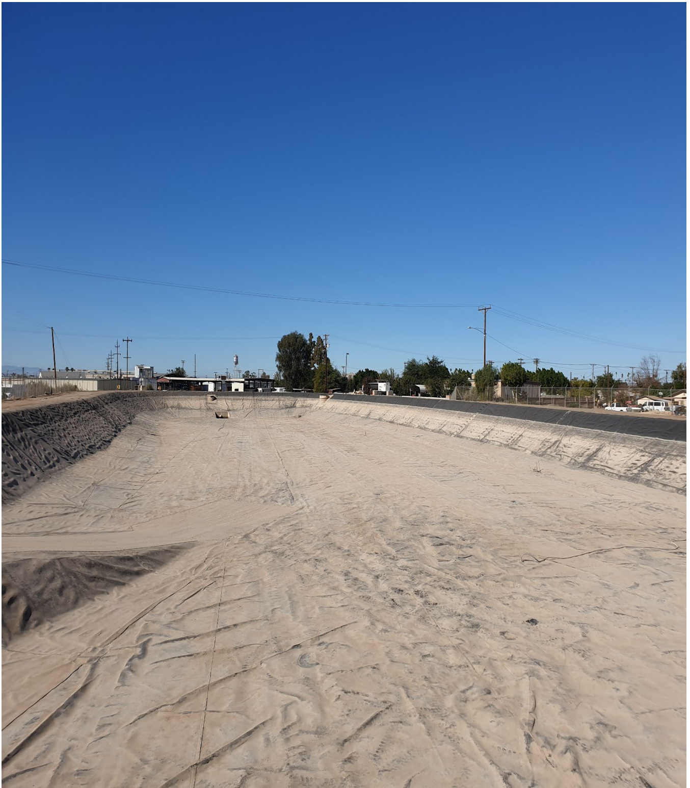
(Pond #3 empty and cleaned ready for patch work by Layfield)
